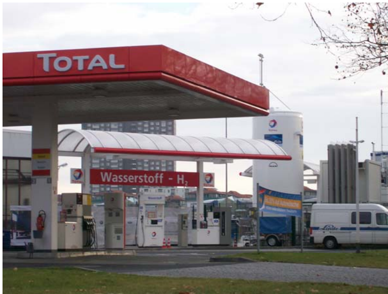
Figure 6: Photograph of public refuelling section of Total multi-fuel station at Berlin Heerstraße [Wurster, 29 Nov. 2007]
